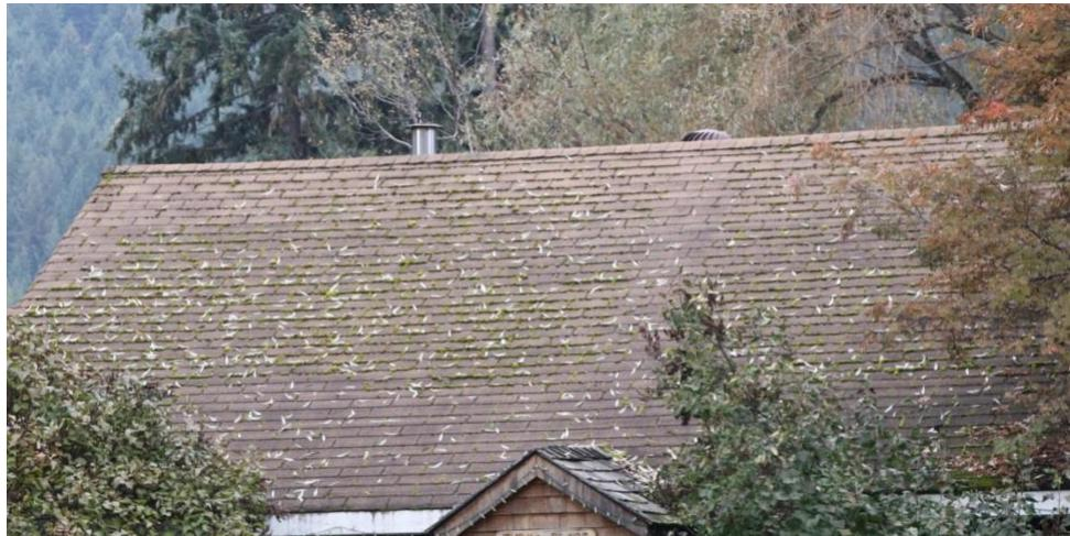
*Figure 8 Aging roofs pose a potential risk to home ignition as the fire-resistant material begins to wear and expose a combustible underside*
