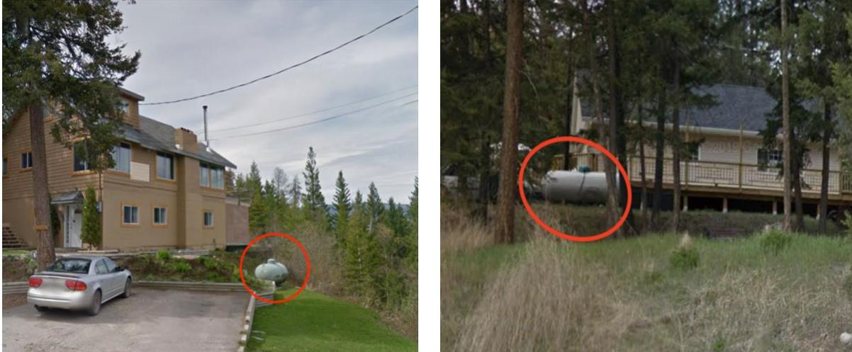
*Figure 11 Propane tanks should be relocated 10m away from a home if possible. There should be a 3m fuel free zone established and relief valves should be tested for functionality and aimed away from structures*
