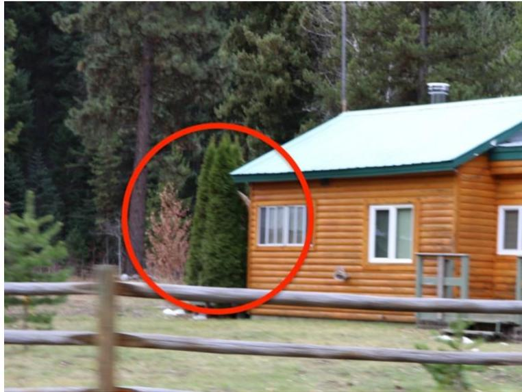
*Figure 9 The presence of nearby combustible debris (such as wood pallets, ladders, building materials etc.) and combustible plants pose a high risk to ignition of a building's exterior.*
