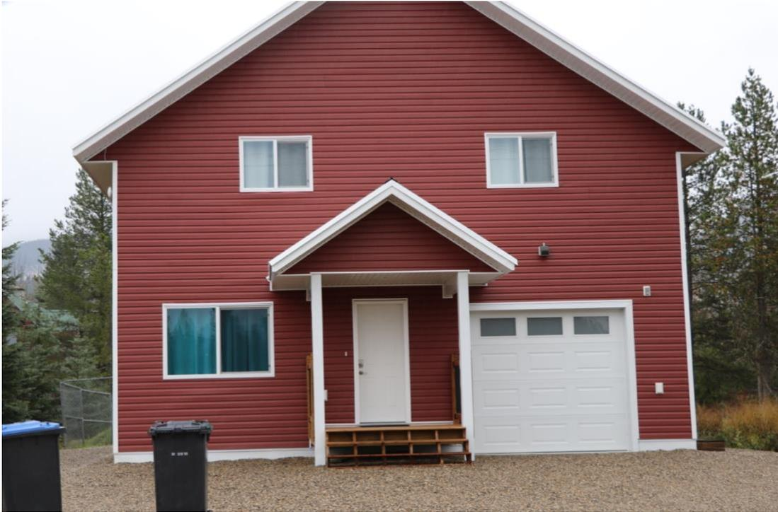
*Figure 7 The presence of nearby combustible debris (such as wood pallets, ladders, building materials etc.) and combustible plants pose a high risk to ignition of a building's exterior. Vinyl siding was the predominant building exterior within the community. This material is highly susceptible to melting and sluffing from extreme radiant heat.*
