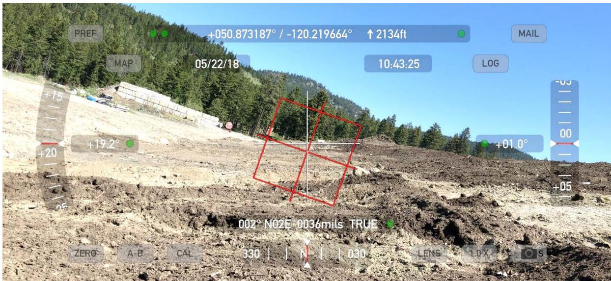
**Photo 4. Proper side slope in Area Slope 4 (3H:1V)**
