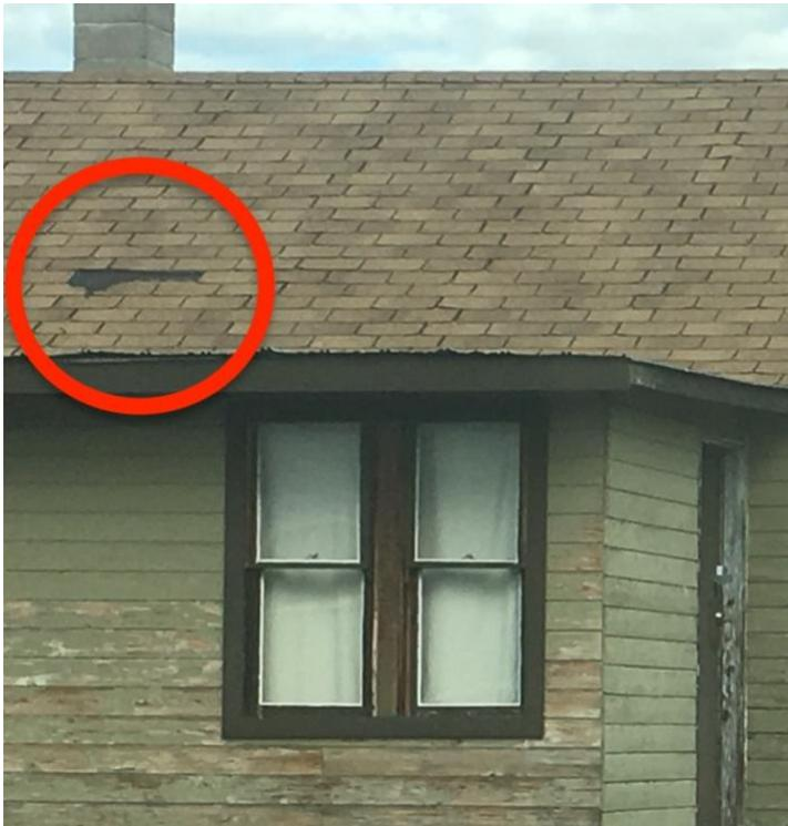
*Figure 8 The roof is one of the most important aspects to the home that can reduce the probability of ignition during a wildfire event. Aging roofs pose a risk to home ignition because of exposures to more readily ignitable materials.*
