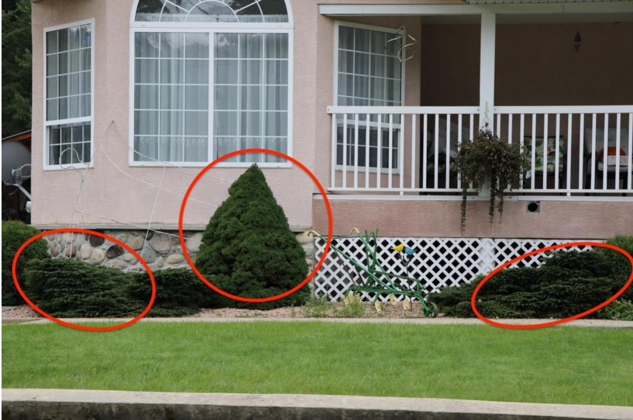
Figure 9 The presence of nearby combustible debris (such as wood pallets, ladders, building materials etc.) and combustible plants pose a high risk to ignition of a building's exterior.
