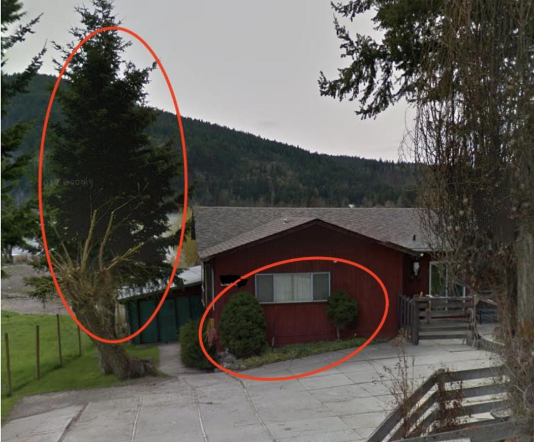
Figure 10 The presence of nearby combustible debris (such as wood pallets, ladders, building materials etc.) and combustible plants pose a high risk to ignition of a building's exterior.
