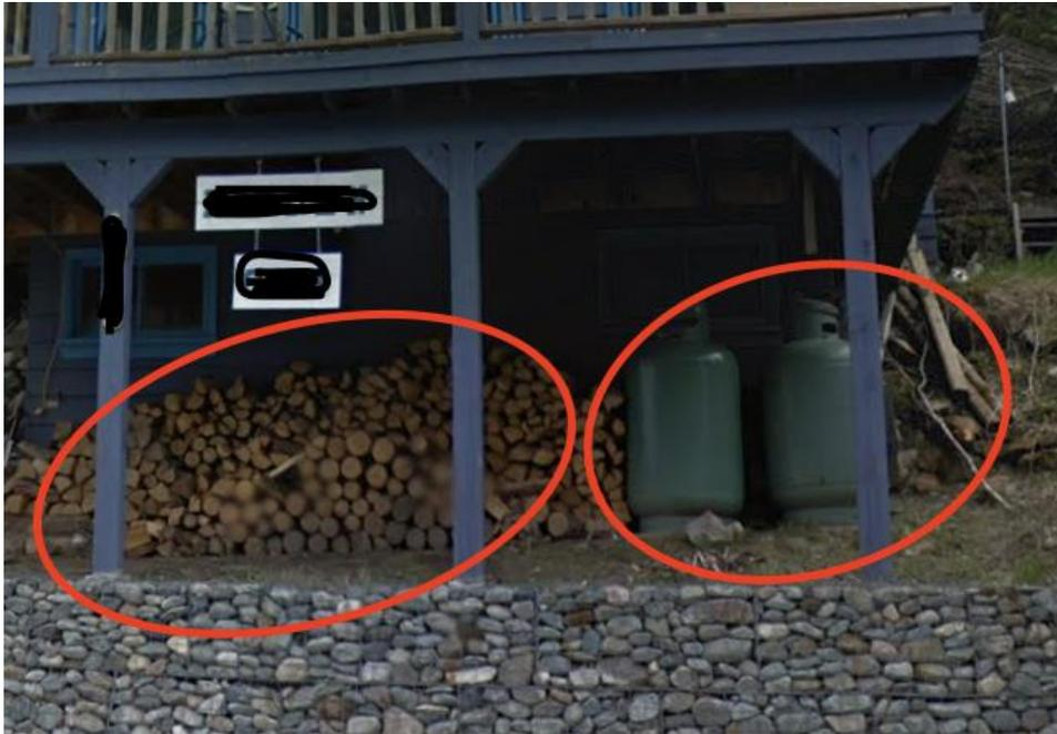
*Figure 8 Firewood and propane tanks should be relocated 10m away from the home - particularly during times of increased threat of wildfire. Firewood has the ability to sustain high-intense heat while propane tanks may explode under extreme radiant heat.*
