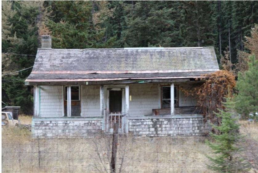
*Figure 12 Abandoned structures, such as this, may be a threat to neighboring structures should it become ignited. Any unmitigated building within 15m of a structure should have FireSmart principles applied – as best as possible – to decrease its risk to ignition and risk to neighboring buildings.*
