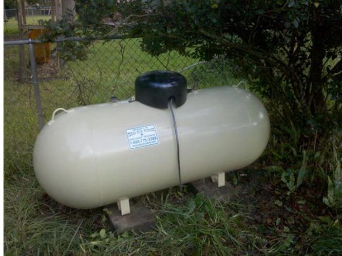
Figure 8 Propane tanks should be cleared of vegetation to mitigate any contact with open flame
