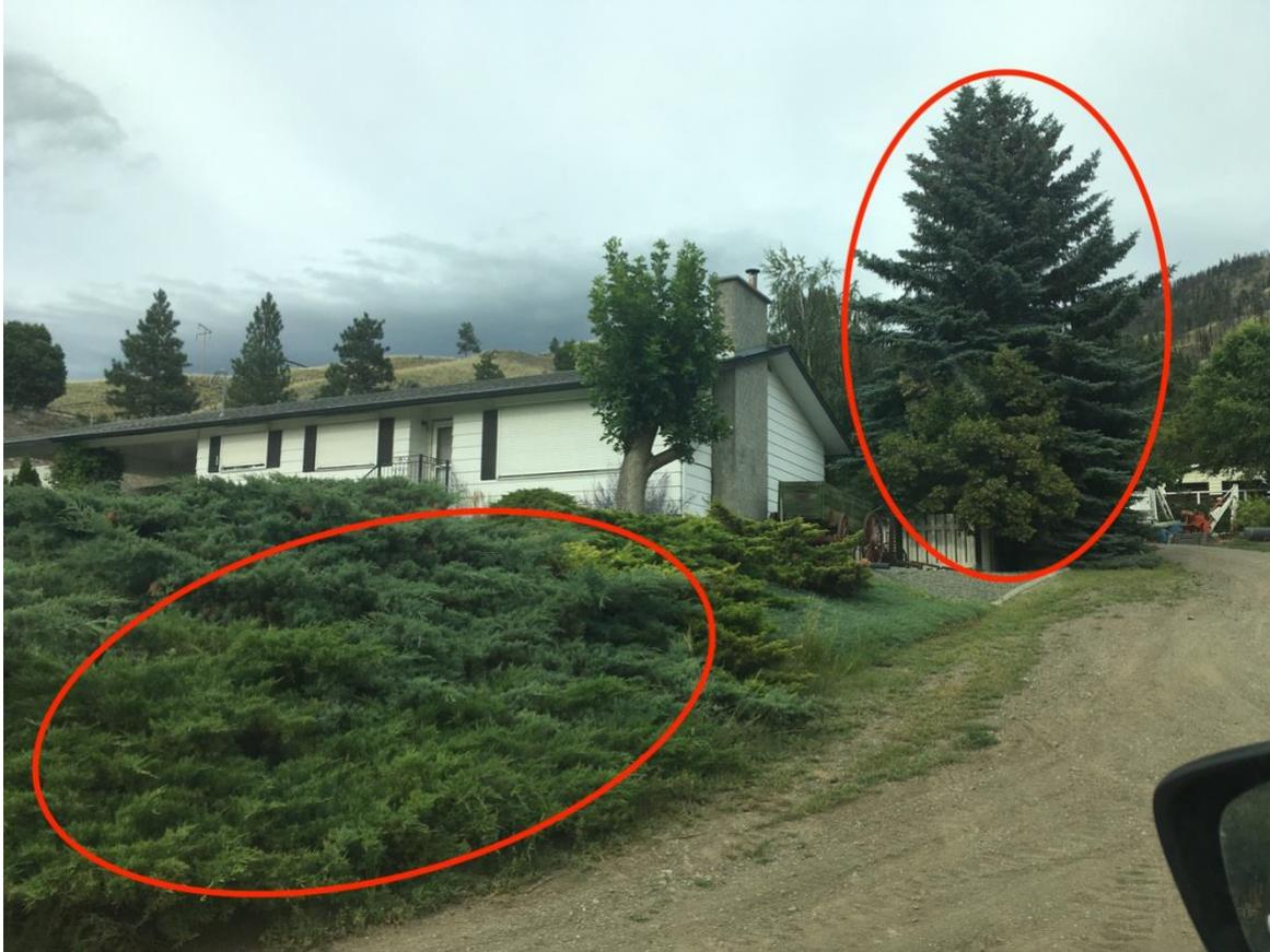
*Figure 7 The presence of nearby conifer vegetation and other combustible plants is a threat to home ignition. They are relatively easy to ignite and will sustain high-intensity heat that will challenge the building's exterior and its resiliency against fire.*
